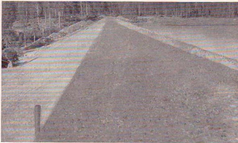
Finished crest of dam, showing rubble-facing on the upstream side.
